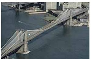
a catenary curve, the natural one made by gravity when a chain is suspended between two points. It has been referred to as the "lazy catenary curve," and is the one made by a hammock. These, made by the four main cables have an effortless ease, and yet each of these cables is capable of supporting 24,621,780 pounds, or 12,300 tons. The daring thrust of the roadway, across what was then the widest span bridged by suspension, is sustained by this effortless curve.
